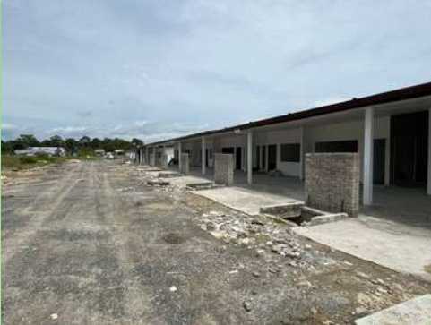
BUILDING WORKS ON-GOING
