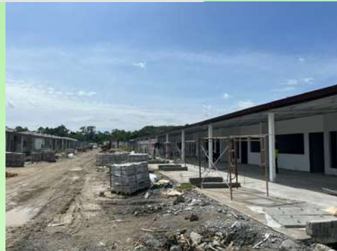
BUILDING WORKS ON-GOING
