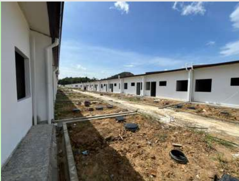
BUILDING WORKS ON-GOING
