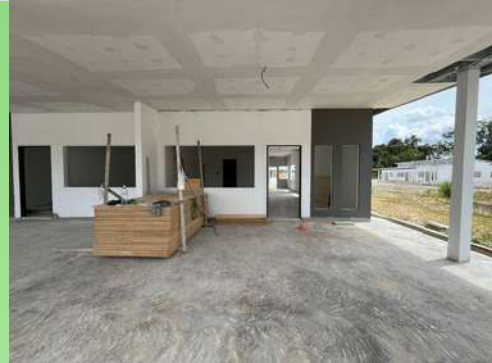
BUILDING WORKS ON-GOING
